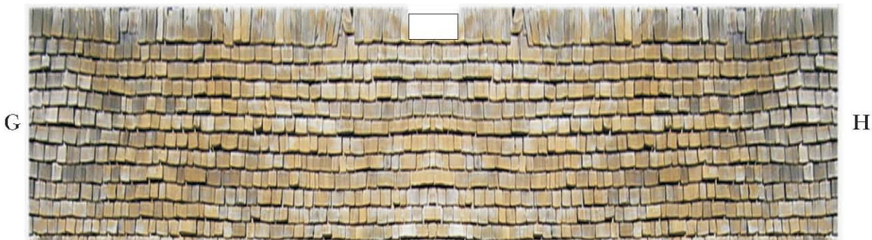
Bottom edge of Front Roof
